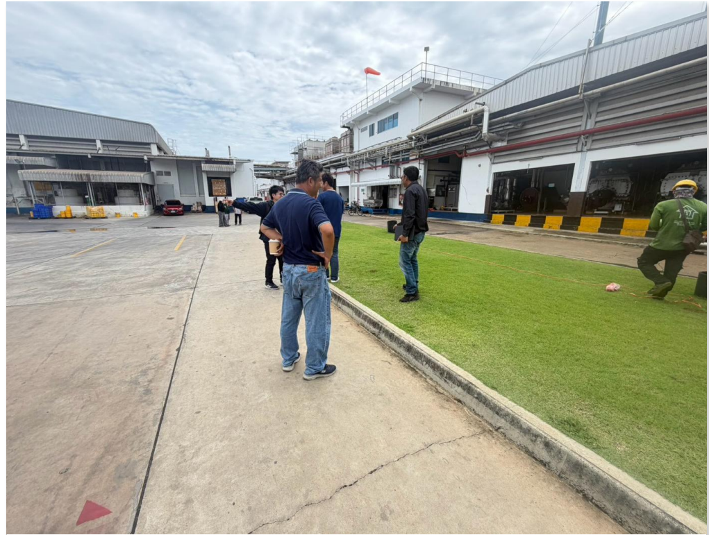
LNG Storage and Regasification Station
